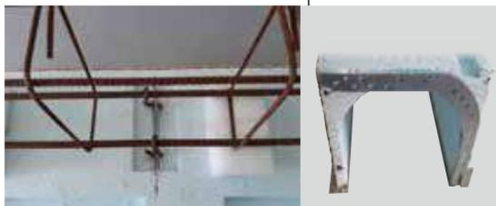
RENFORT DANS COFFRE PERMETTANT DE REPREDRE LE CHAÎNAGE
